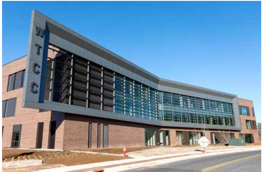
Wake Tech's new campus strengthens connections to RTP business and industry.
